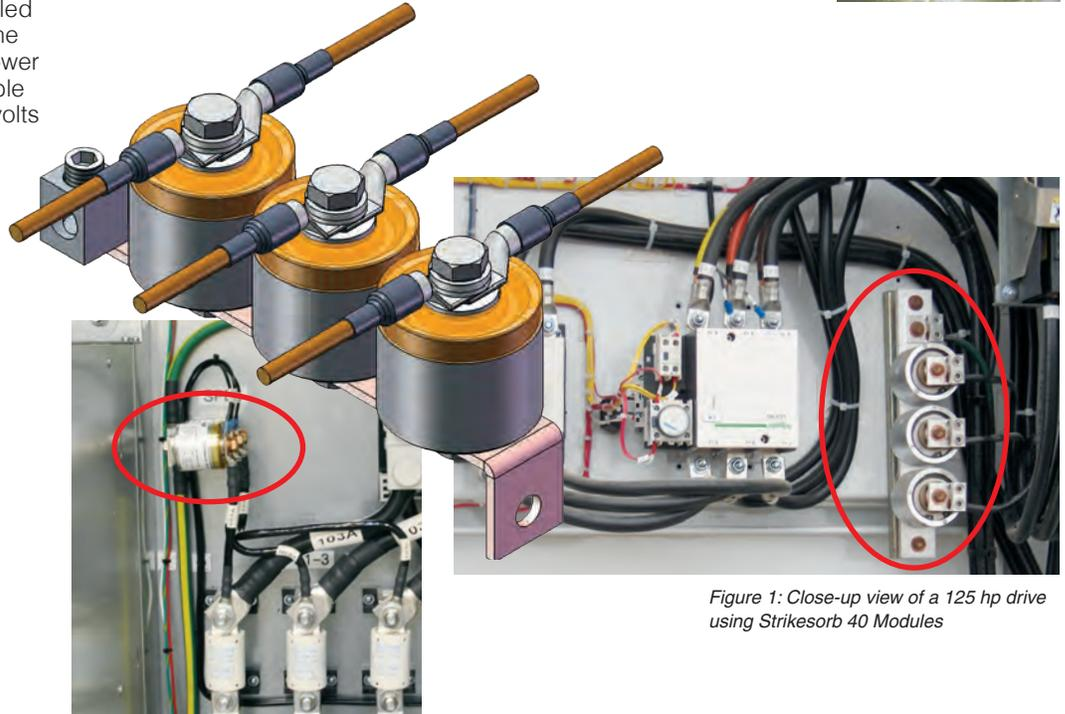
Figure 1: Close-up view of a 125 hp drive using Strikesorb 40 Modules
