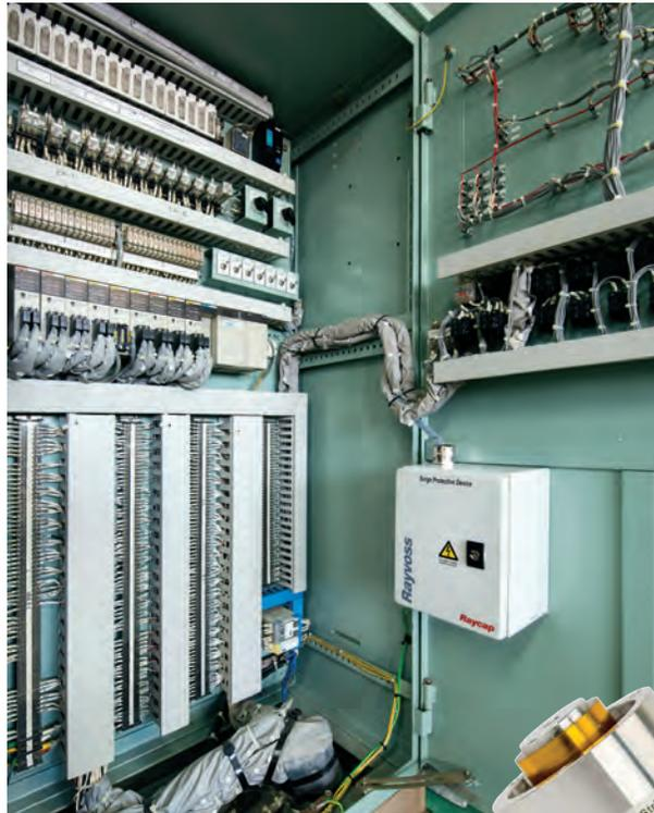
Figure 2: Rayvoss M surge protective device installation on the inert gas control panel.
