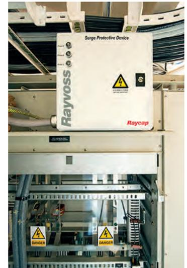
Figure 3: Rayvoss M systems strategically placed at the Emergency Switch Board (ESB) of the vessel provides vital protection to critical shipboard functions.
