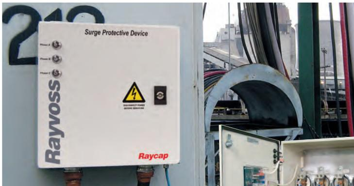
Rayvoss installed on a conveyor belt
